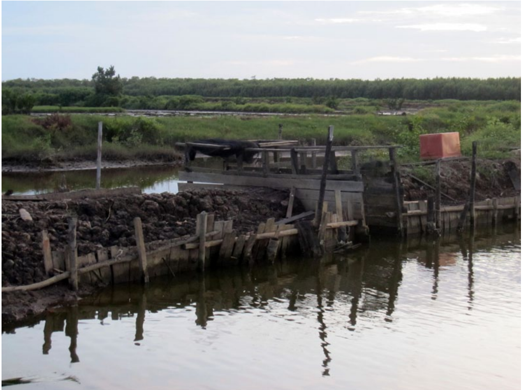
Fig.7: Sluice gate of an aquaculture pond on Sepuk Laut Island (S. Karstens, 2012)
