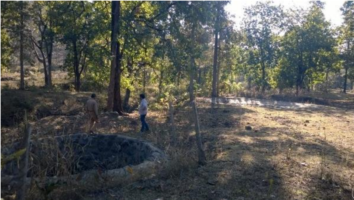
Picture 24 - Well and water storage structure built for animals in Parasda village, Bhaura range, Betul
