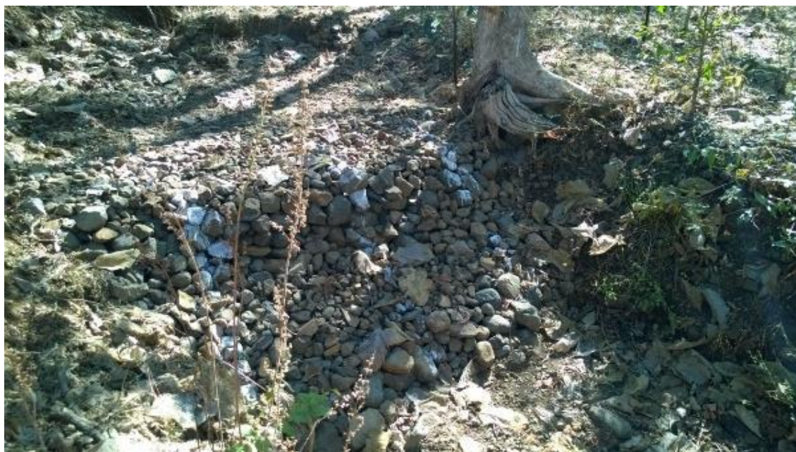
Picture 19 – Loose boulder check dam in Dukarsela village, Ambada range, Chhindwara
