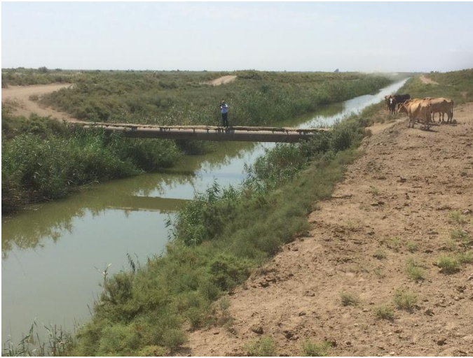
Photo: The old and not safe passage of the main canal.
