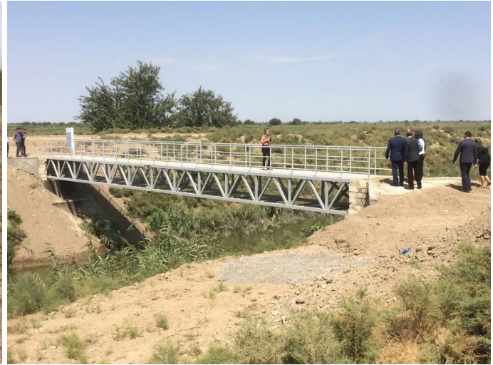
Photo: The newly constructed passage.
